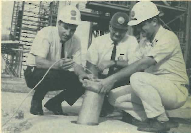
Pan American engineers removing a pressure gauge from its earth well to check it out prior to launch. Author Golub is at left.
