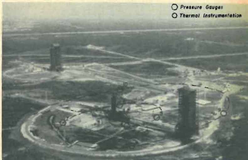
The over-all view of Launch Complex 36 at Cape Kennedy with the location of the pressure gauges and thermal sensors indicated.
